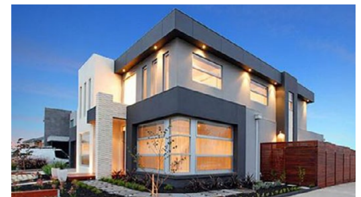
Figure 3. Facade wraps around the corner
